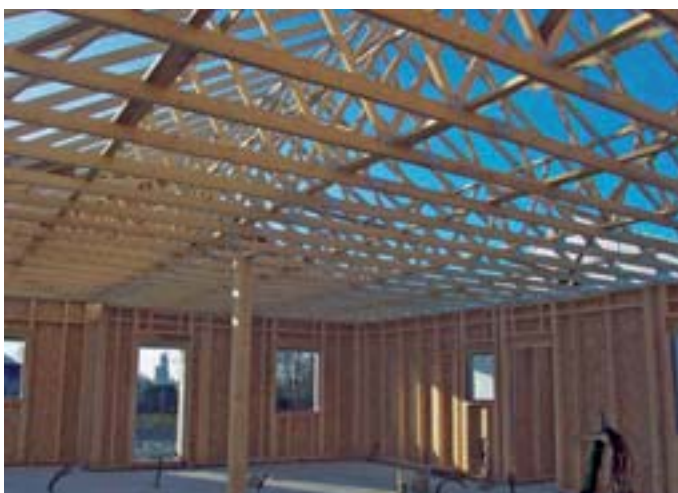
Charpente Industrielle (Source FCBA)
